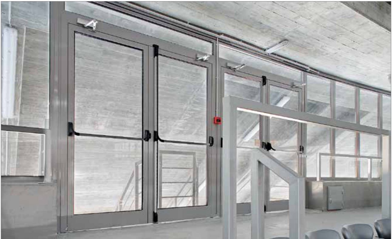
Sports Hall, Zadar, Croatia (Photo: Robert Les)
