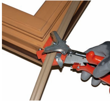
Cut the weatherseal in position
