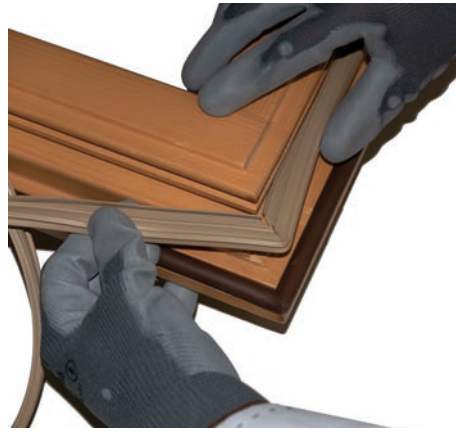
Insert the weatherseal
