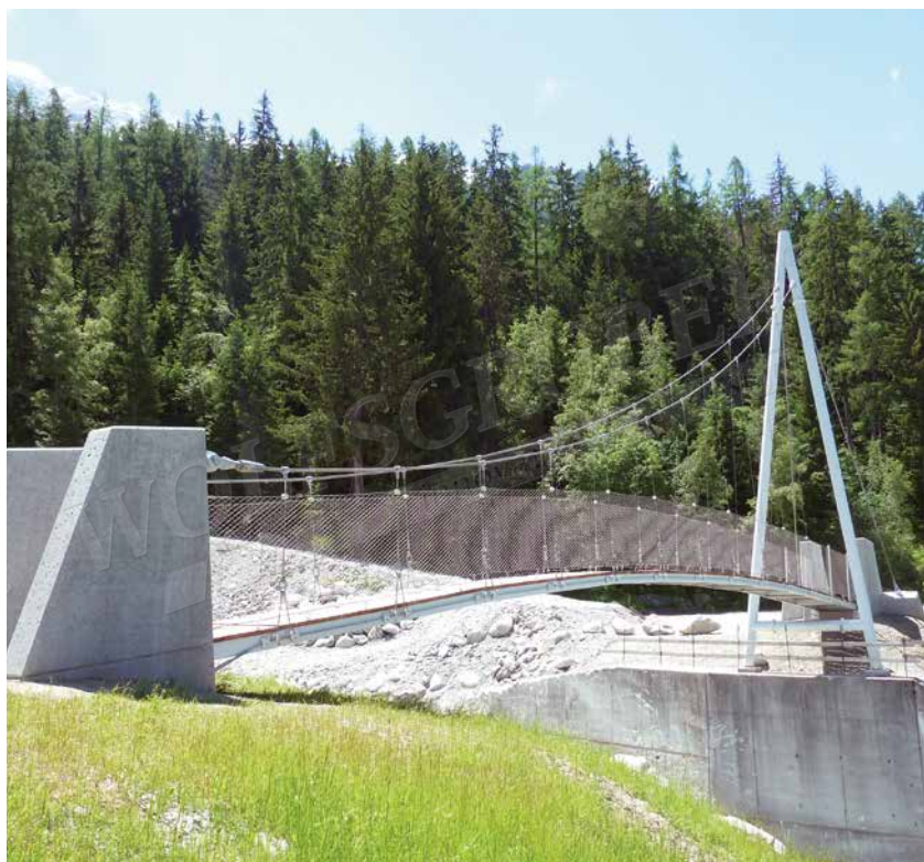
X-TEND 95 m 2 , \diamond 60 mm, \varnothing 2 mm
