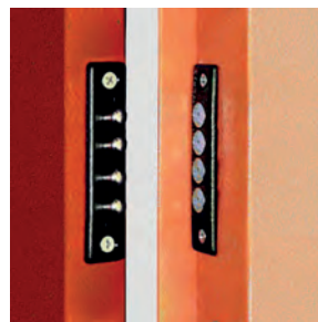
Electrical contacts between leaf and doorframe
